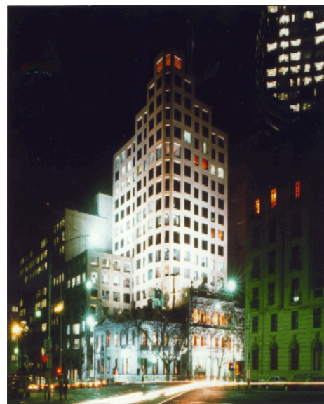
No. 1 Collins Street, Melbourne
